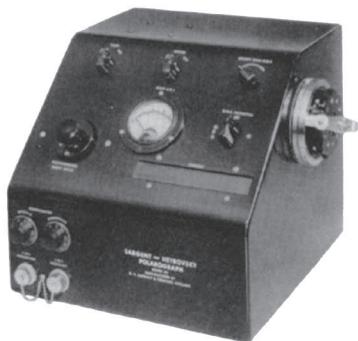
Figure 6. Photographic recording polarograph from E. H. Sargent & Company (model XI).
